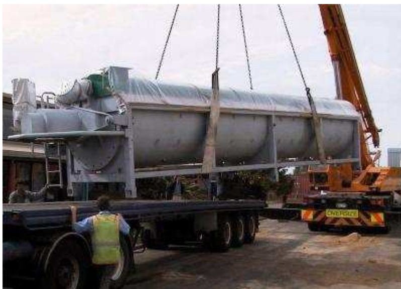
Figure 100: Installation of HotRot at Sewage Treatment Works in New Zealand.
