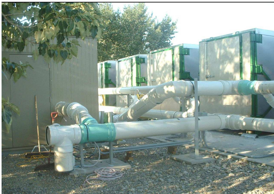
Figure 111: The Aeration System of the CV Composter at Okotoks
