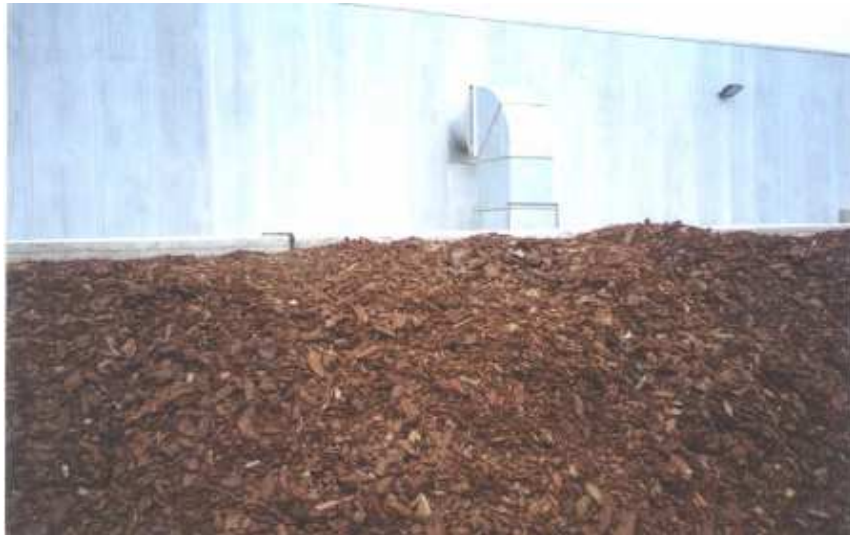
Figure 96: Biofilter in the Composting Plant of Botarell
