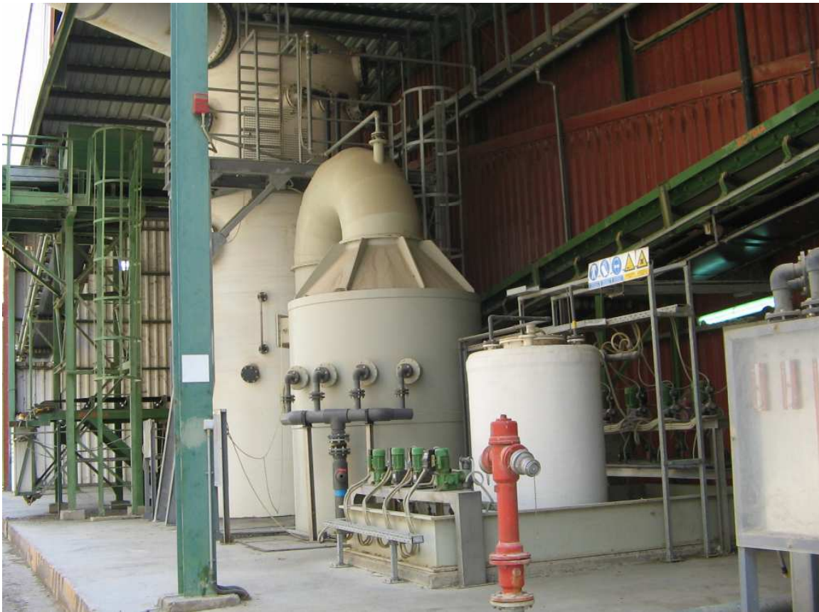
Figure 15: Scrubbers Employed for Air Treatment
