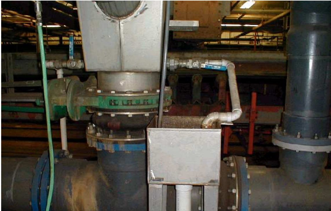
Figure 74: Collection of Excess Water ‘Squeezed out’ from Sewage Sludge
