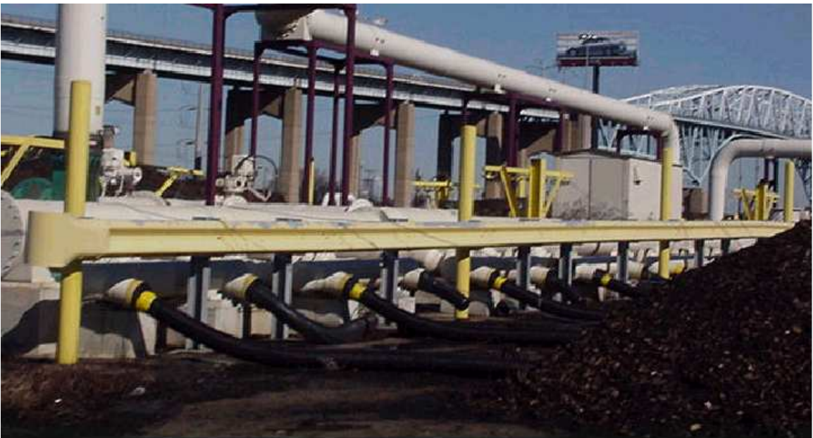
Figure 82: Perforated Pipe Underneath the Composting Mix.
